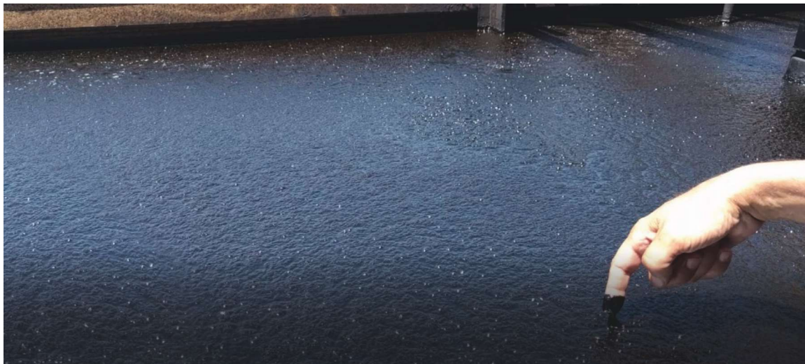
Oil collects on the surface of a Nano Gas treatment tank. (Photo courtesy of Nano Gas Technologies Inc.)
